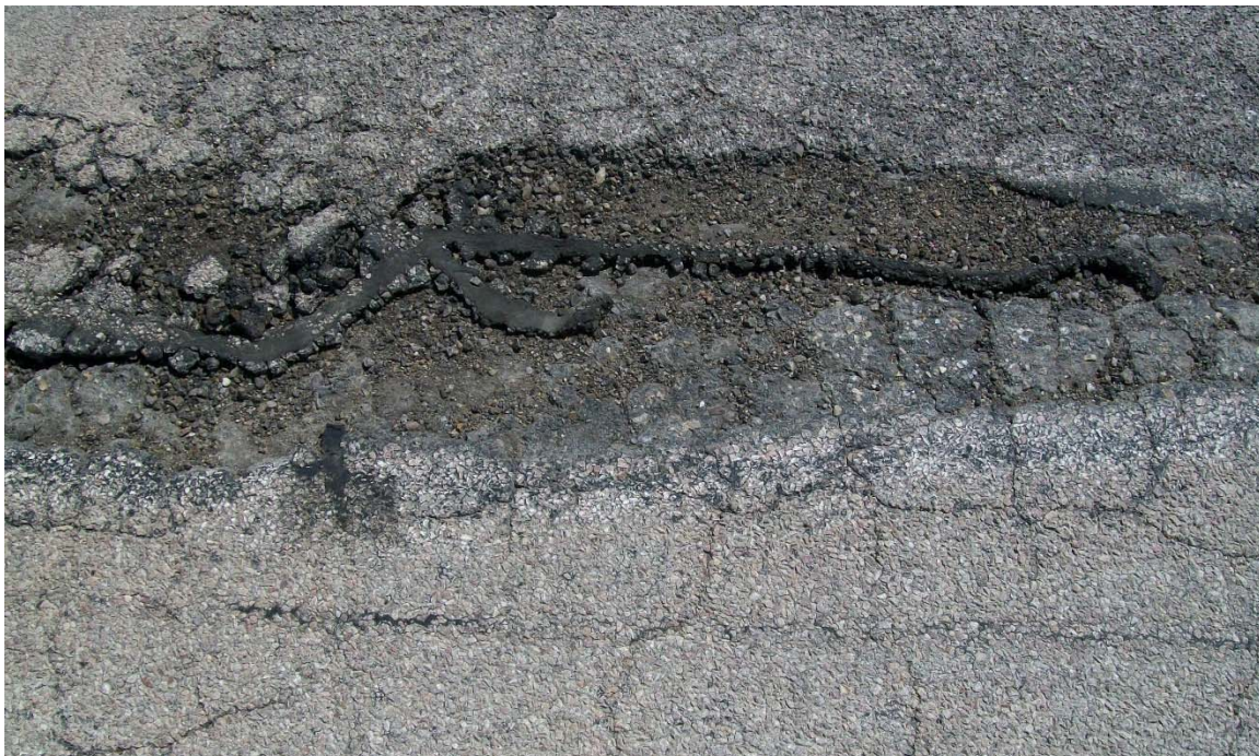
Asphalt breakups along the project route
