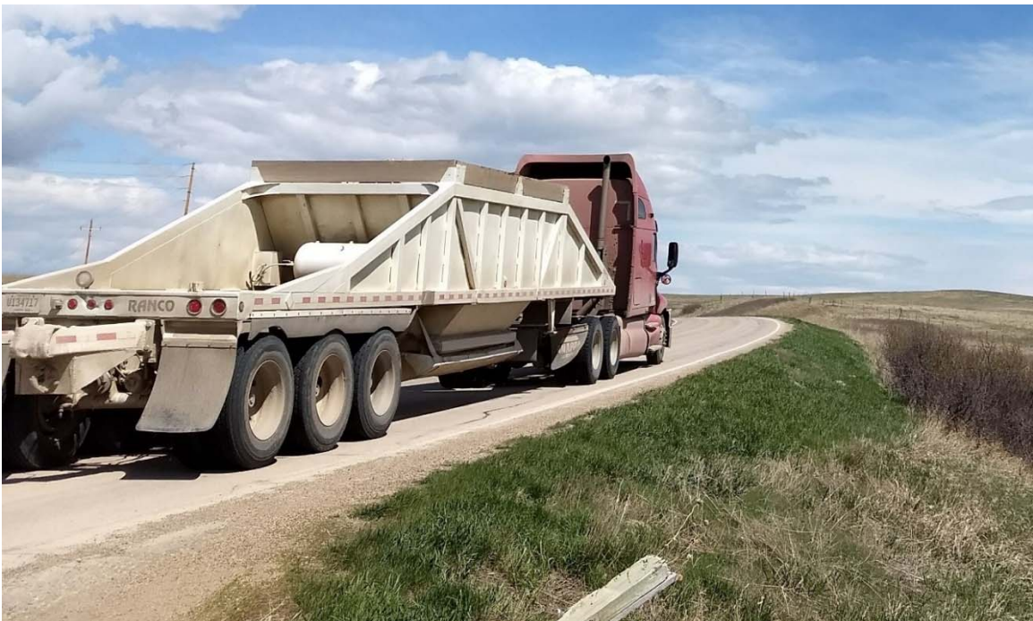
The existing roadway cross section and geometry does not support truck traffic. Most locations where trucks enter the project route do not have sufficient sight distance.
