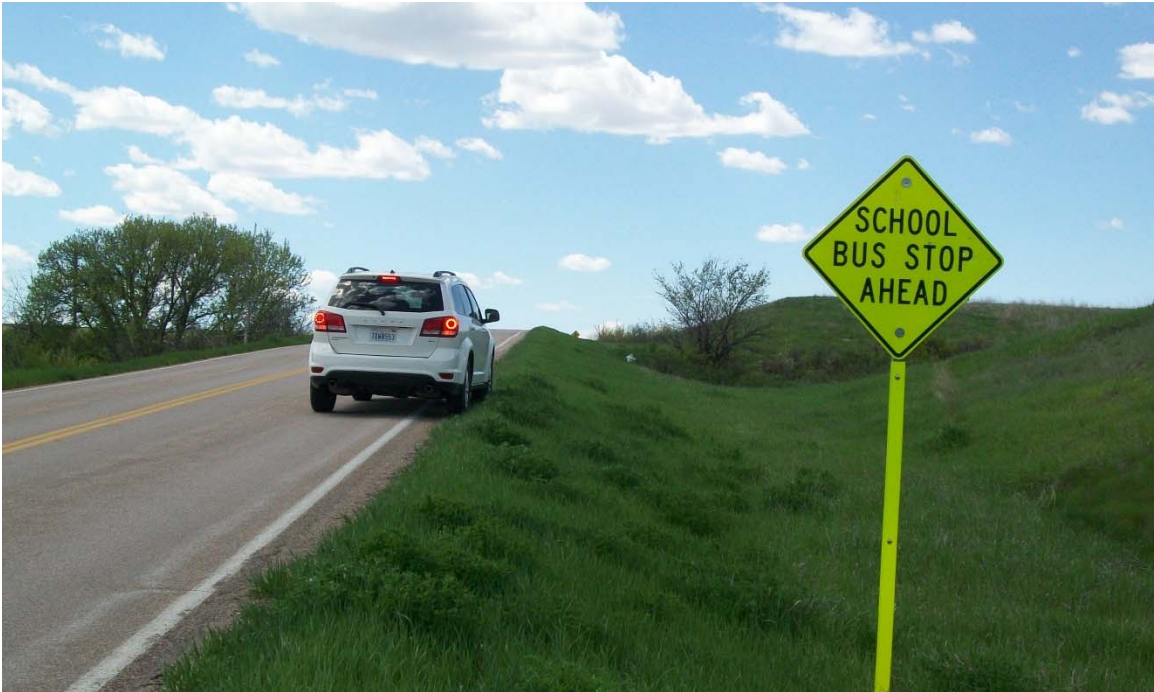
School buses make several stops along the project route. Buses stop in roadway lane due to no shoulder and steep sides slopes.
