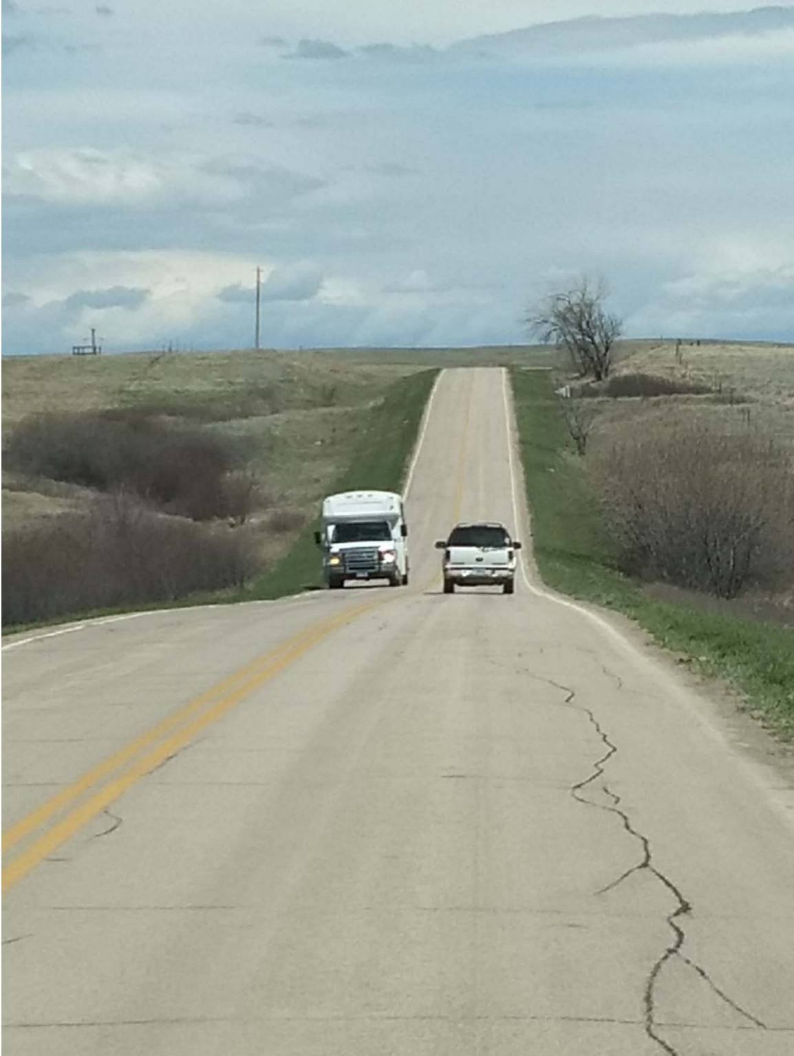
Narrow roadway for transit buses. Bus is driving on edge line.
