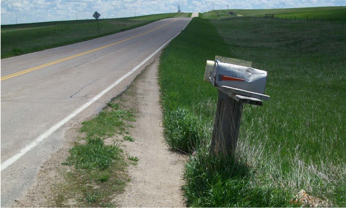
Existing mailboxes do not have breakaway bases and mail carriers must stop in roadway to deliver mail.
