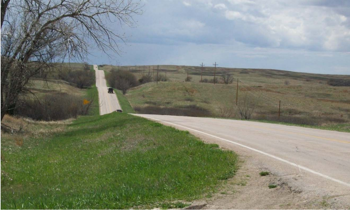
Excessive vertical curves
