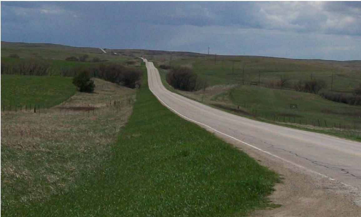
Excessive vertical curves
