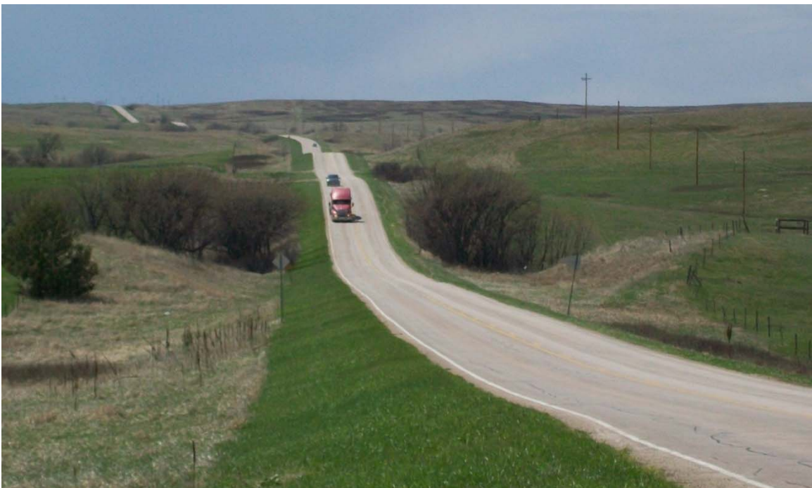
Narrow roadway with truck traffic
