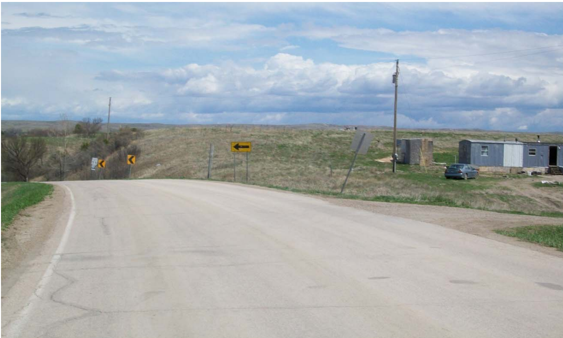
BIA 2 – looking east at compound horizontal curves and vertical curve
