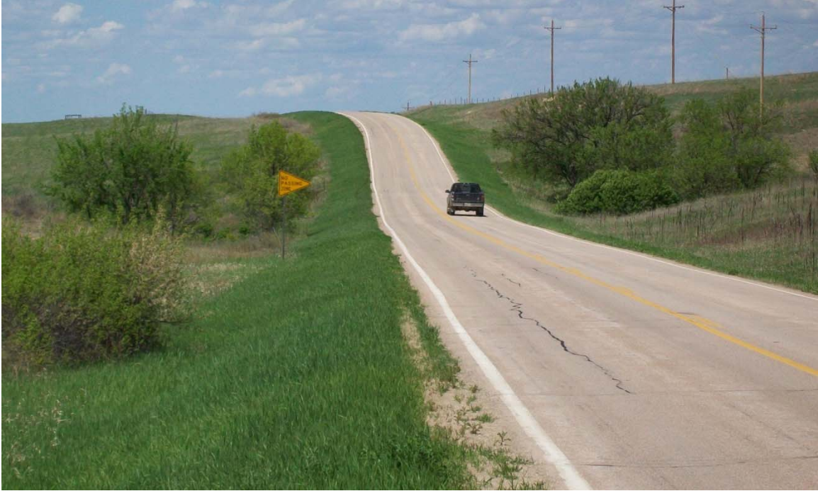
A sharp horizontal curve begins at the vertical curve crest.
