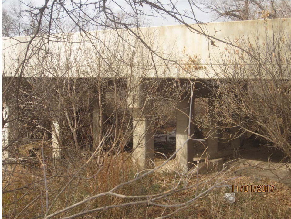
View North Through Bridge Looking Downstream
