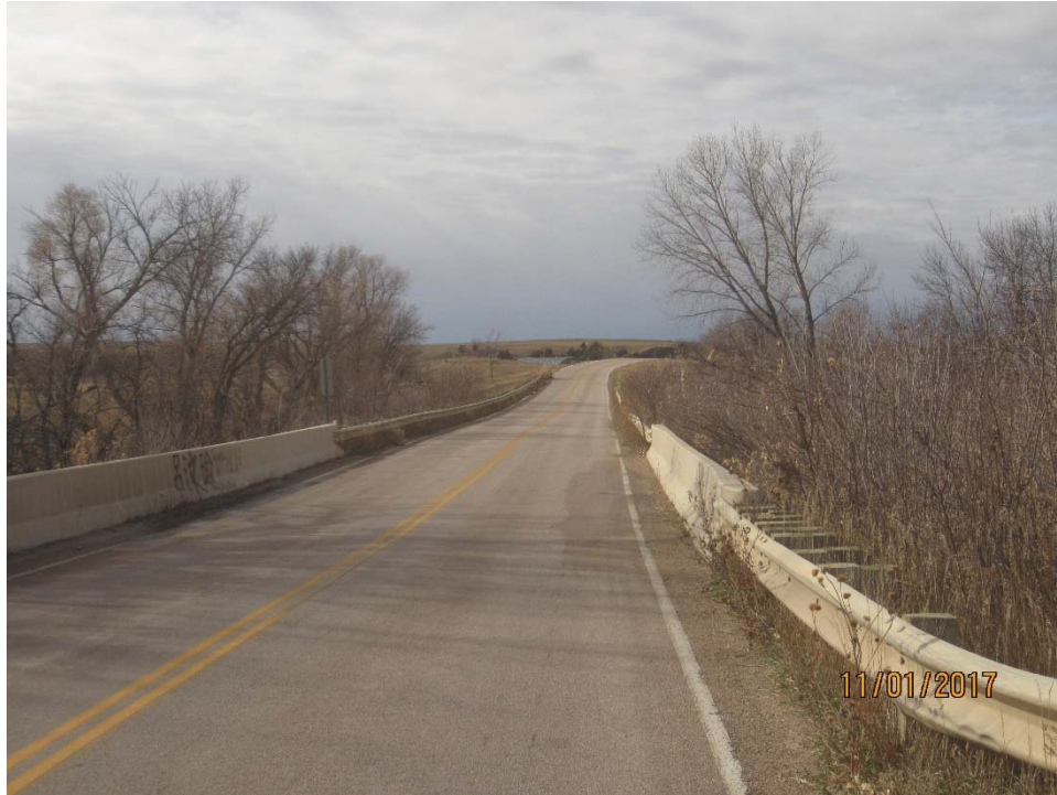
View of bridge looking west
