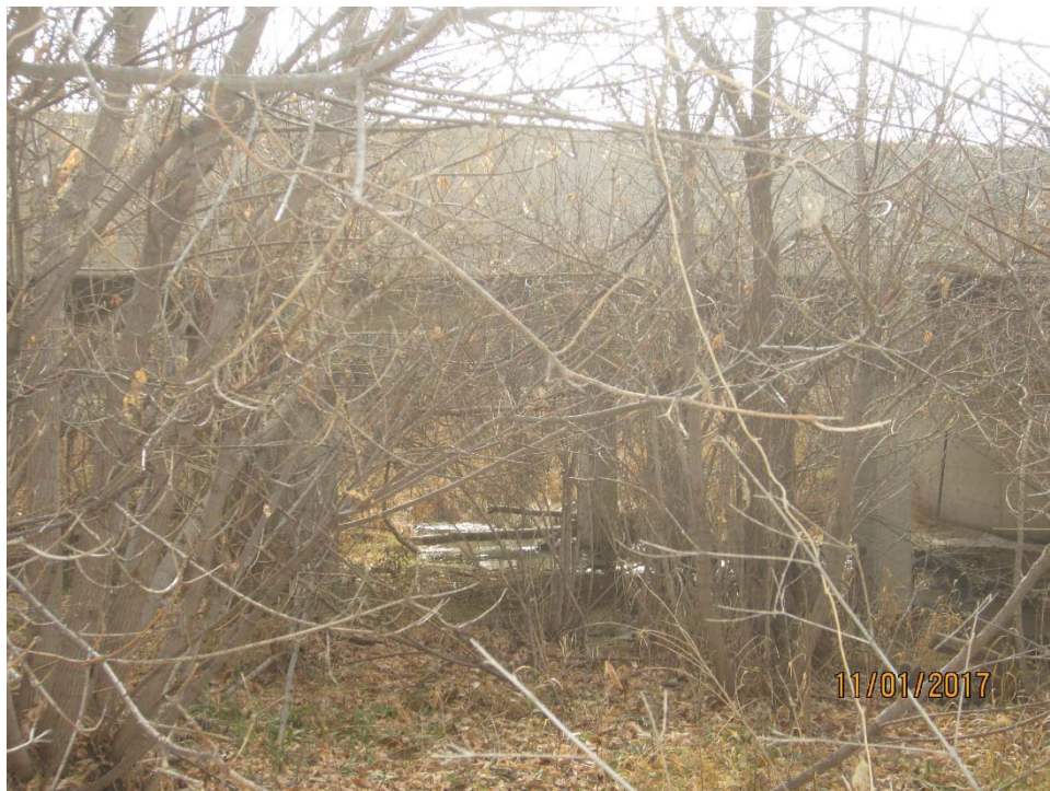
View South Through Bridge Looking Upstream
