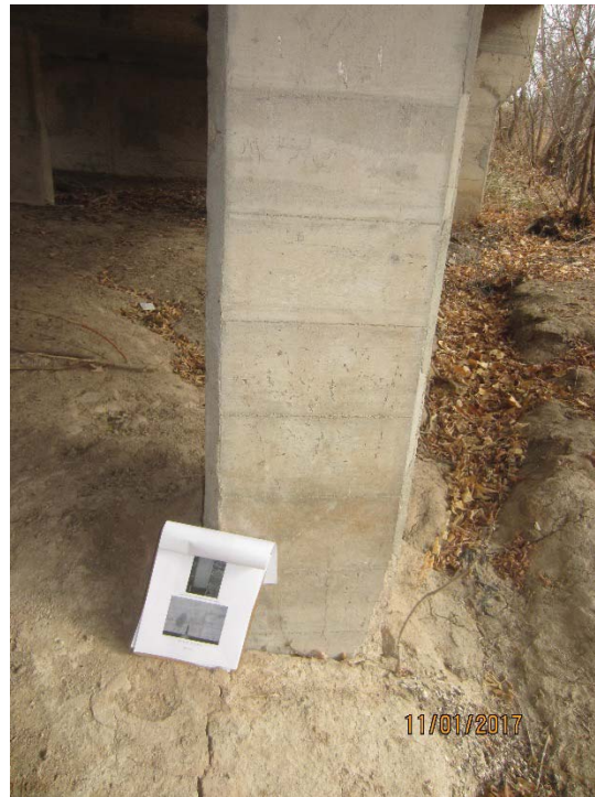
Typical pier column condition
