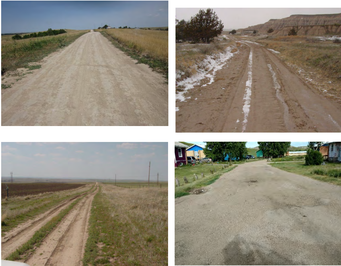
FIGURE 3-10 - Non-Paved Roadway Types and Conditions
