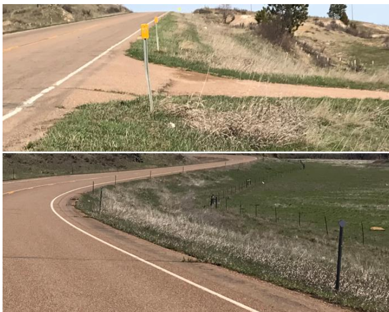
Figure 5.7: Roadside Delineators Example
