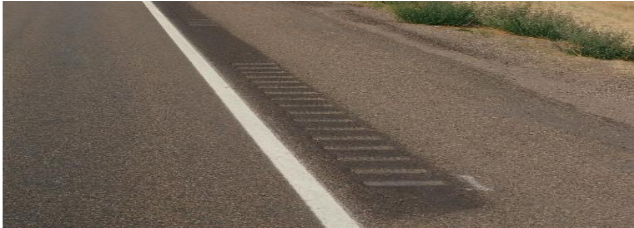
Figure 5.6: Shoulder Rumble Strips
