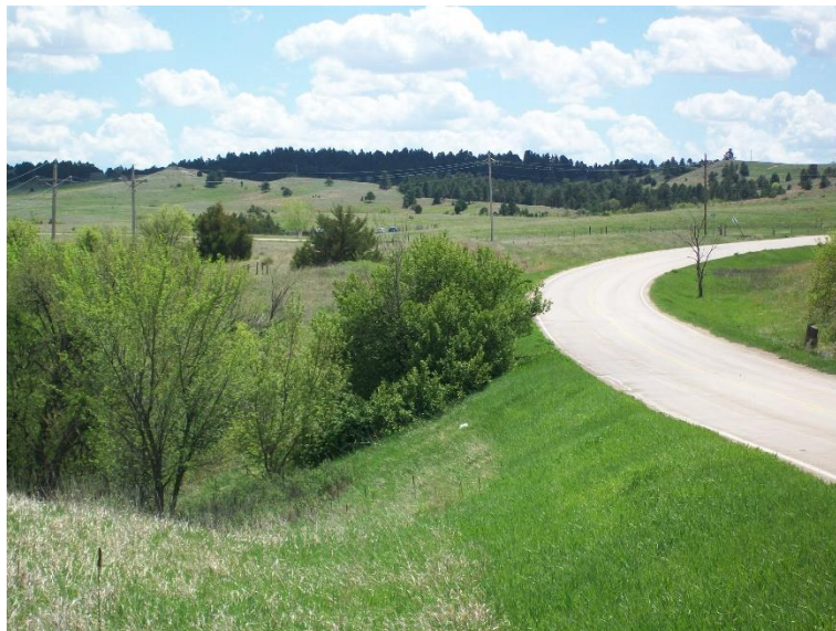
Figure 5.10: Sharp Horizontal Curve
