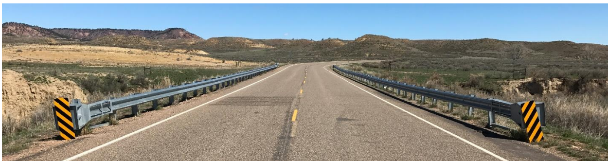
Figure 5.5: Guardrail Installed for Steep Side Slopes
