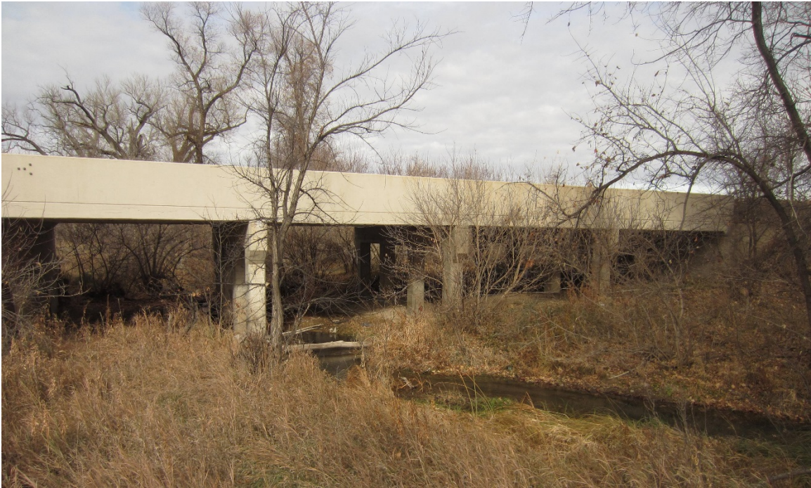
Potato Creek Bridge - Profile
