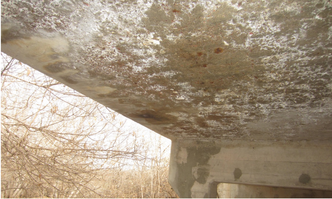
Potato Creek Bridge – Under Deck
